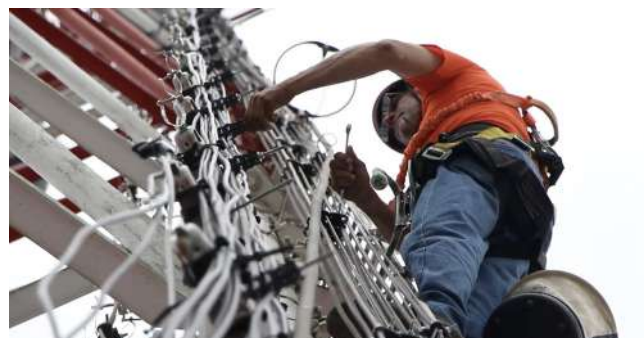
Our +Móvil technician maintaining phone and broadband connection in Panama.
