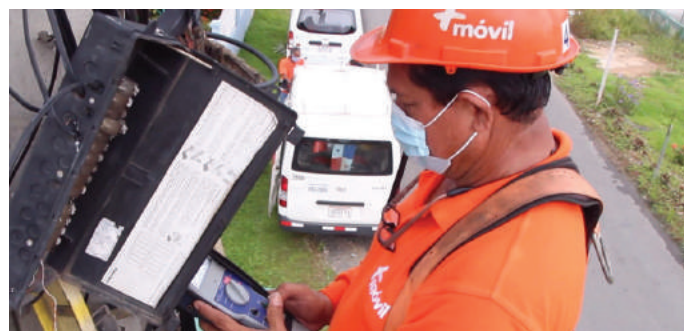
Our Cable & Wireless Panama technician in the field working to keep our communities connected
